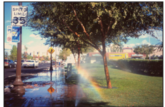
Figure 2 - Sprinklers out of adjustment.
