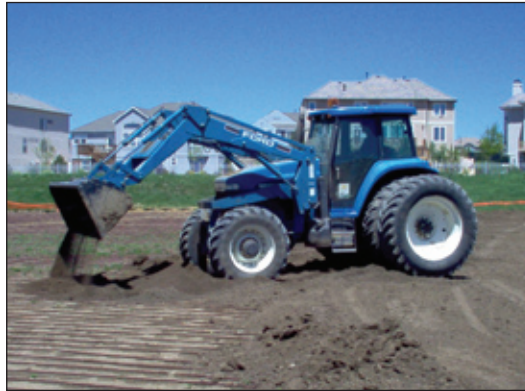
Figure 34 - Subgrade installation of Techline CV with soil being laid over a grid layout. Note how the loader is moving parallel to the dripperlines to minimize the rows from shifting.
