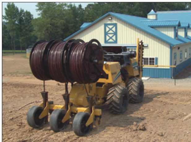
Figure 31 - A Vermeer® LM42 laying Netafim dripperline three rows at a time.
