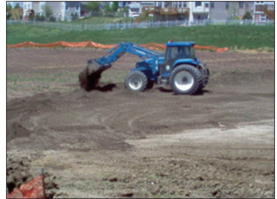
Figure 34 - Subgrade installation of Techline CV with soil being laid over a grid layout. Note how the loader is moving parallel to the dripperlines to minimize the rows from shifting.
